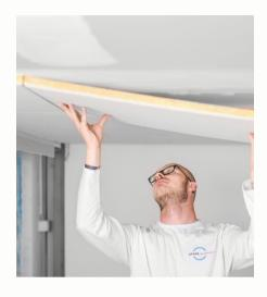
**2. Adhering the acoustic panels** The acoustic panels are easily applied to the substrate with an adhesive. For curved surfaces the panels are cut and prepared accordingly on site.
