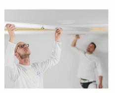
**1. Preparing the surface** BASWA systems can be glued directly onto concrete or suspended substructures (mineral substrate).
